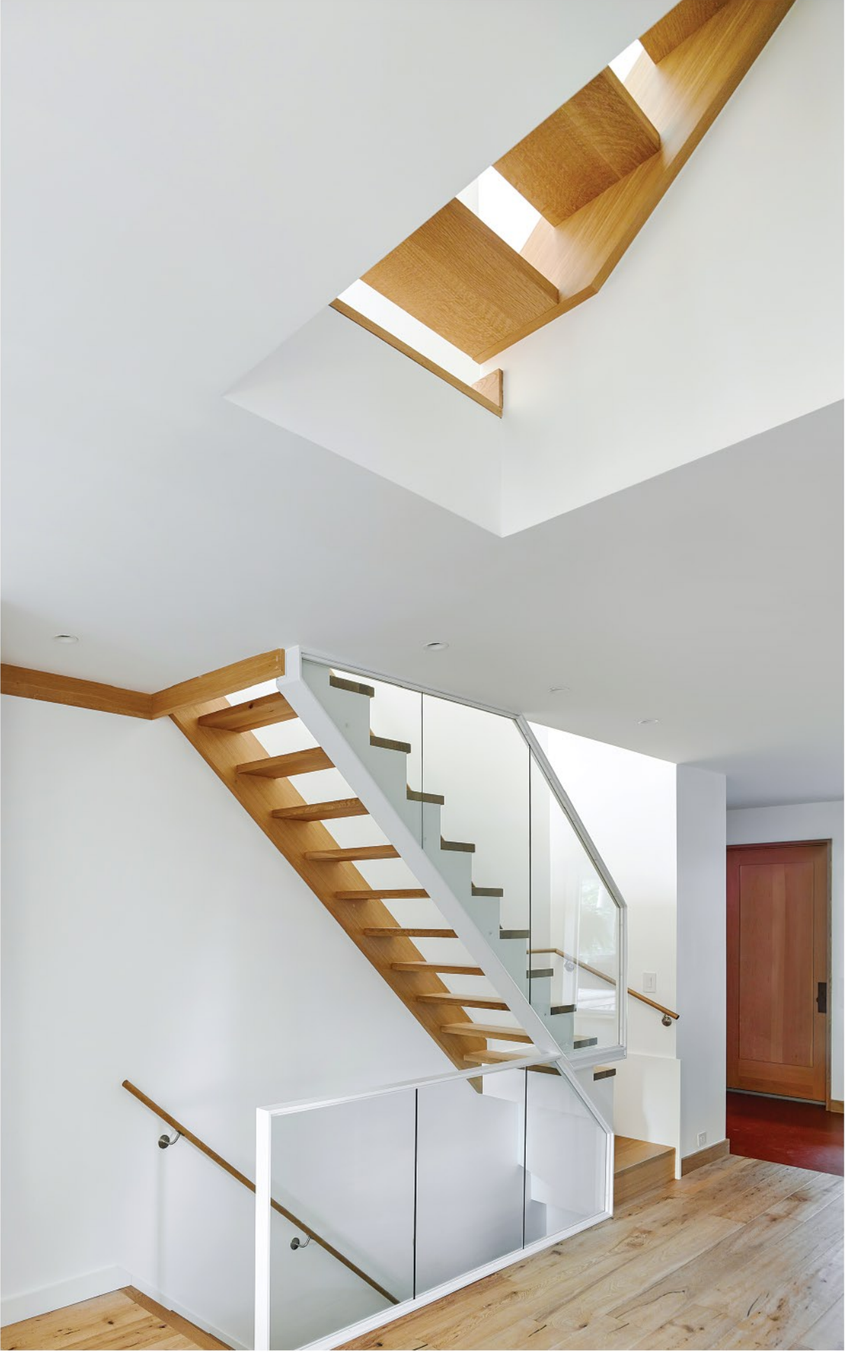
LEFT The staircase (built by LaFabrika) spans three storeys and features open white oak treads on concealed brackets. Neue Floors' white oak planks run throughout. CENTRE Red Forbo Marmoleum flooring is used in high-traffic areas, like the entry. The custom Douglas fir bench was built by Derek Nicholson. Windows and doors by Marvin. RIGHT A rectangular opening above the custom kitchen (by BL Woodworking & Design) allows light to pour through the house via the open risers of the stairs. Pendants from Progress Lighting.
